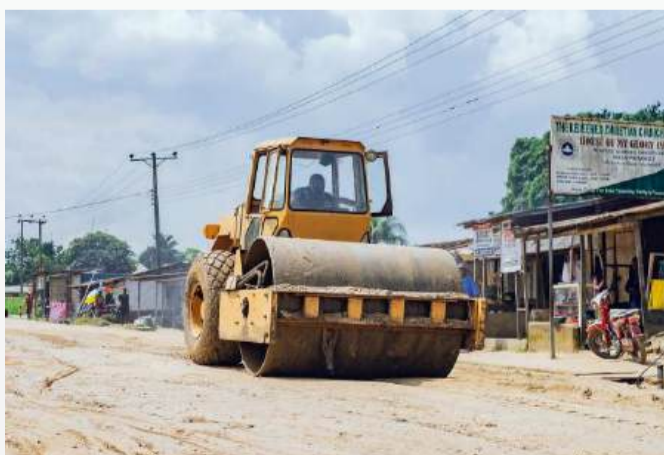
Road Rehabilitation projects across communities in Obigbo
