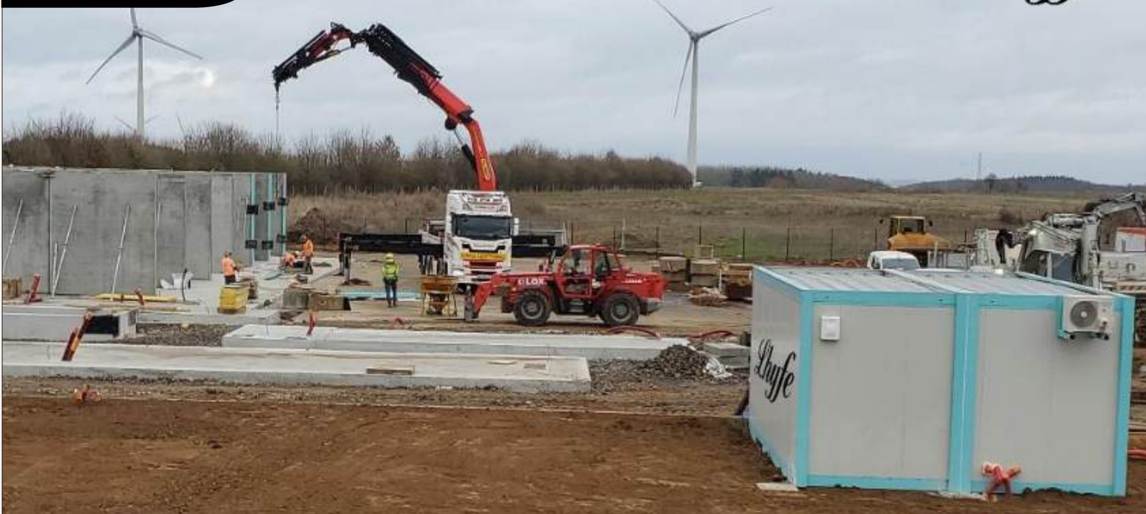
Image: civil engineering work in progress at the Lhyfe site in Croixrault (France)
